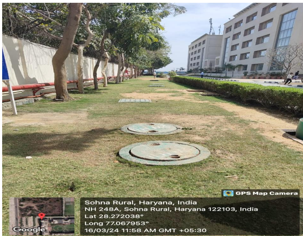
Rainwater Harvesting Pits at K.R. Mangalam University, Sohna — constructed to collect and recharge rainwater into the groundwater table, promoting sustainable water conservation practices
