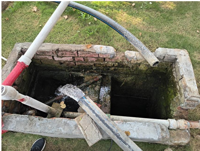
Groundwater extraction and recharge inspection point at K.R. Mangalam University
