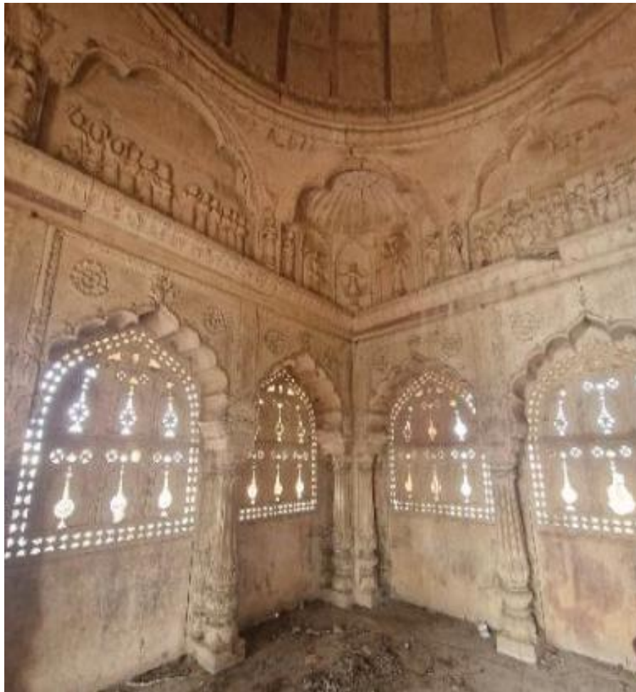
Fig.8: Perforated jali screens enabling cross-ventilation Source- Author
