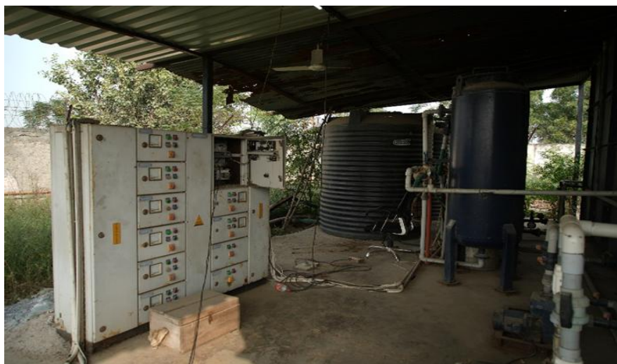
100,000 L/day STP at K R Mangalam University treating wastewater for reuse in irrigation and green landscaping
