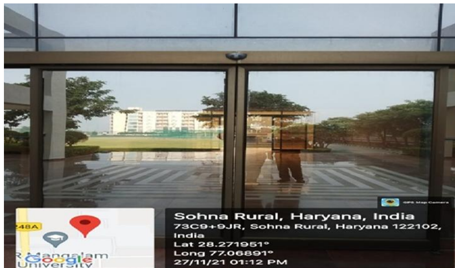
Automated sensor-operated entry doors reducing conditioned-air loss & improving building energy efficiency
