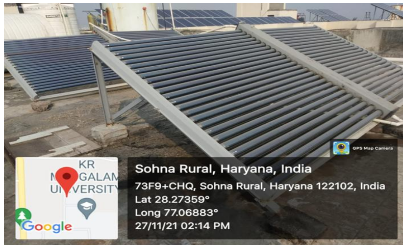
Solar thermal system providing hot water in hostels, reducing LPG and grid energy dependence
