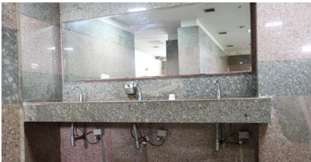
Sensor Taps in the Washrooms of the University to reduce water wastage
