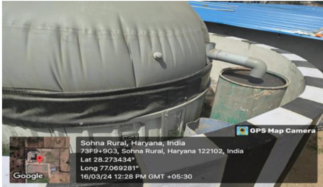
Biogas outlet & slurry discharge used as organic manure for campus horticulture sustainability
