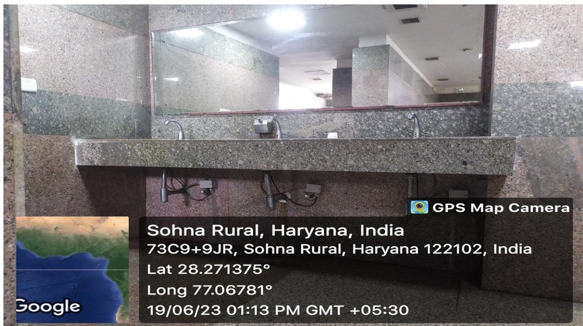
Water-efficient washbasins installed at K.R. Mangalam University, Sohna — equipped with sensor-based taps to minimize water wastage and promote responsible water usage across campus
