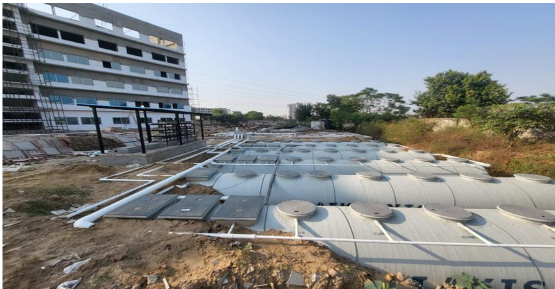
Sewage Treatment Plant (STP) at K.R. Mangalam University, Sohna — designed for efficient wastewater treatment and reuse for landscaping and non-potable purposes
