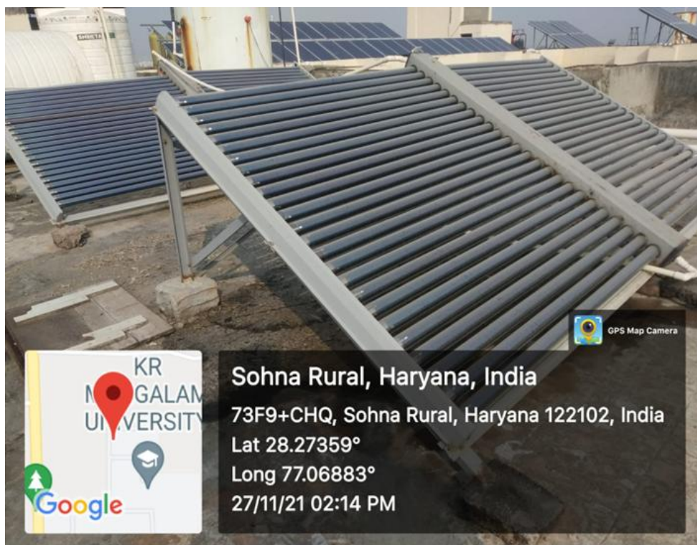
Solar thermal system providing hot water in hostels, reducing LPG and grid energy dependence
