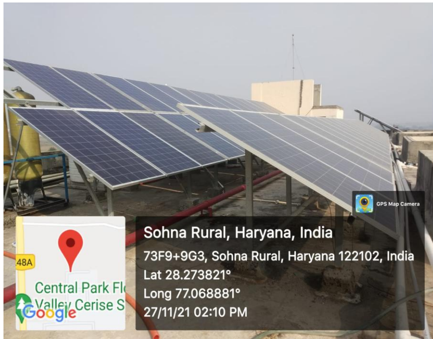
310 kWp rooftop solar PV system across Academic Blocks and hostels, generating clean electricity and reducing dependence on grid power
