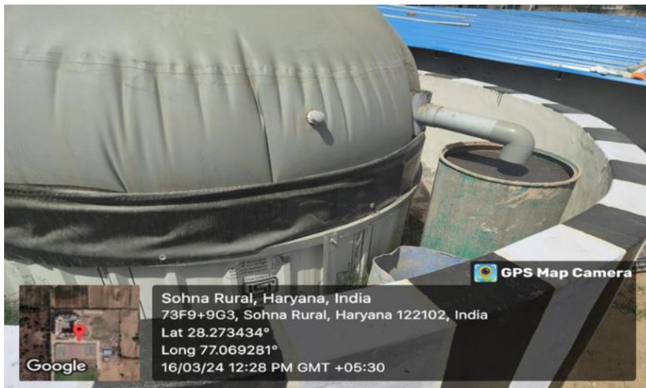
Biogas outlet & slurry discharge used as organic manure for campus horticulture sustainability
