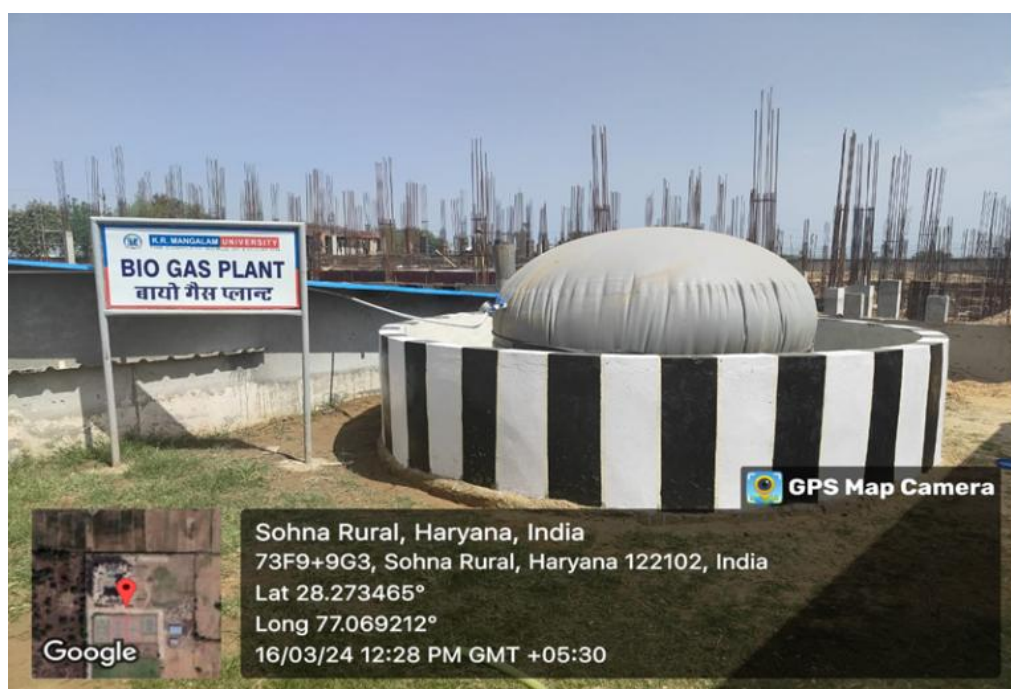
Campus biogas plant converting food waste into clean energy, replacing LPG & generating organic fertiliser
