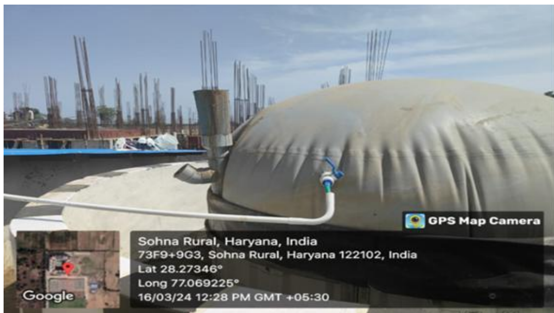
Campus biogas plant converting food waste into clean energy, replacing LPG & generating organic fertiliser
