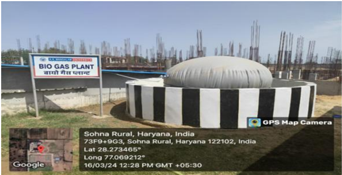
Campus biogas plant converting food waste into clean energy, replacing LPG & generating organic fertiliser
