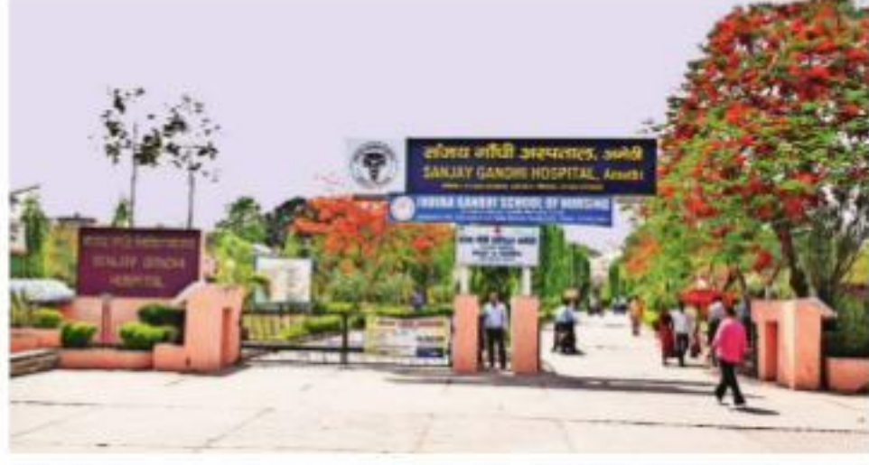
The 100-bed hospital has been in operation in Munshiganj of Amethi since 1989. File
